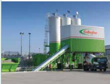
mixer with two loading points. With three 80-tonne silos, the plant has the capacity to produce large pours in excess of 200m<sup>3</sup>. Most of the aggregates will come from the company's Hermitage Quarry near Maidstone.
