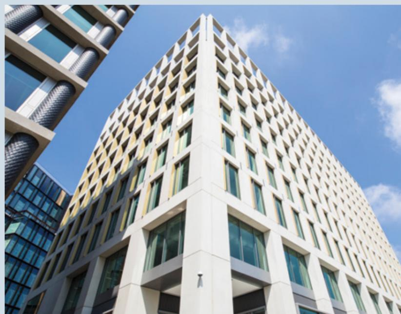
Two Pancras Square: concrete panels incorporate a system to collect and divert rainwater for use within the building
