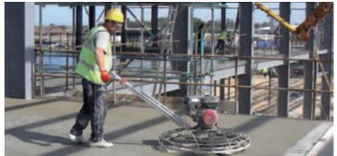
*Figure 14. Power trowelling for a hard wearing finish.*
