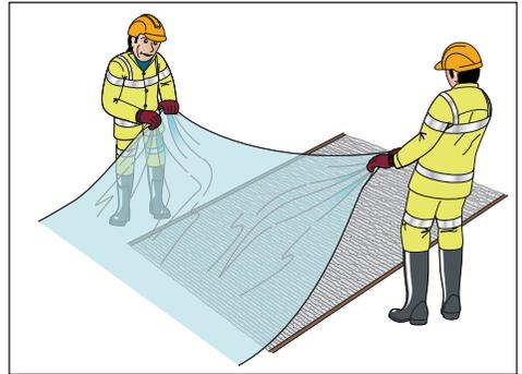
**Figure 15.** Polythene sheeting used to protect concrete.
