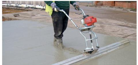
*Figure 13. Petrol powered single beam screed*
