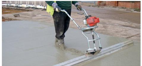
*Figure 13. Petrol powered single beam screed*
