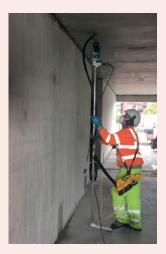
There is often a need to drill holes into the underside of concrete floors to allow false ceiling, pipework and services to be hung. Frequently precast hollow core floor beams need to be drilled to release water trapped in the cores.
