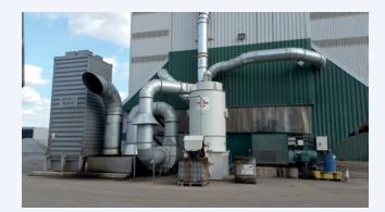
The system extracted fumes and dust from the mixed material storage bins and the vehicle loading bin area. Extractions fans capable of a maximum volume flow of 28,000m<sup>3</sup>/hr were used. The captured emission dust and fumes were processed through a wet scrubber, which removed heavier particles, and then a carbon filtration system to remove nuisance fumes.
