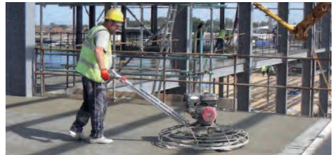
Figure 14. Power trowelling for a hard wearing finish.
