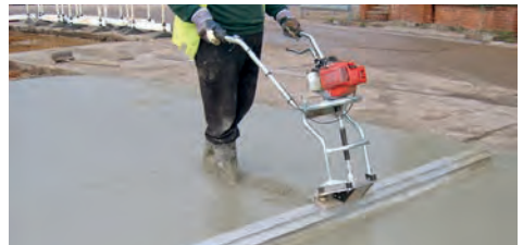
Figure 13. Petrol powered single beam screed
