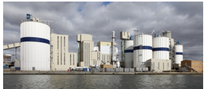
Continued investment in new plant such as this cement blending plant in east London has helped reduce CO 2 emissions by cutting back clinker production
