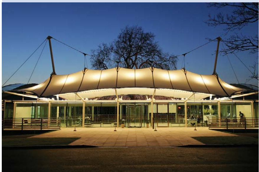
Roehampton indoor tennis arena – built using ground granulated blastfurnace slag
