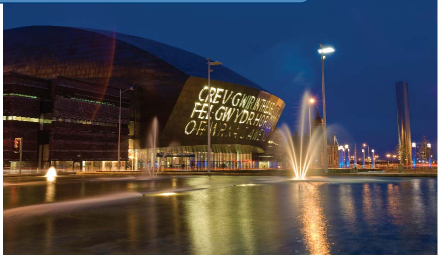
The Welsh Assembly building in Cardiff – built using ground granulated blastfurnace slag
