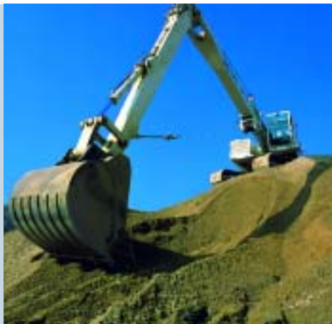
Pumping is needed to allow many sites to be worked dry
