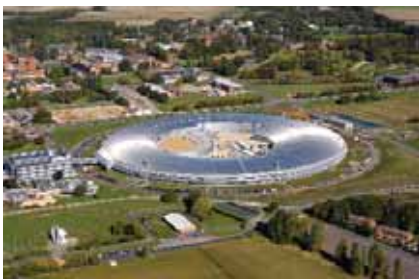
The Diamond Light Source synchrotron is a new scientific facility on the Harwell Chilton science campus in South Oxfordshire. It can be described as a series of 'super microscopes' and is housed in a futuristic doughnut-shaped building which covers the area of 5 football pitches. It will ultimately host up to 40 cutting edge research stations, called beamlines, supporting the life, physical and environmental sciences. Over 35,000m 3 of concrete were supplied during its construction.
