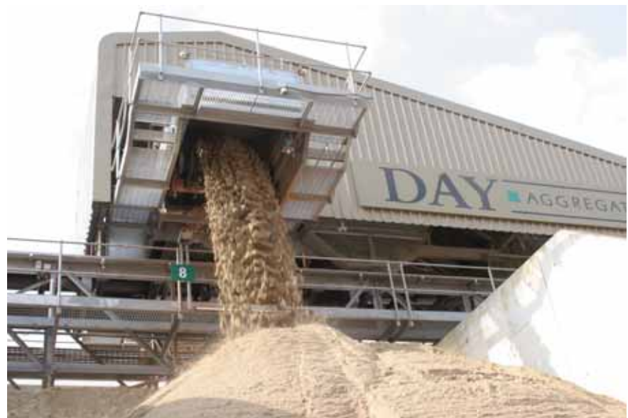
Day Aggregates is creating high-quality blends of primary and recycled aggregates at its site at Purley in the south of London. The rail-delivered primary aggregate is blended with construction waste from building sites all over London. The computer-controlled mixing process creates blends using anything from five per cent to 60% recycled materials.
