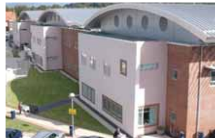
Great Western Hospital, Swindon. One hundred new hospitals will have been built in the UK between 1997 and 2010.
