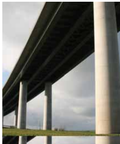
This £100 million bridge to the Thames estuary island of Sheppey will overcome traffic chaos associated with the current bridge, which has to be raised around 20 times a day for ships to pass. The structure has required 59,000 tonnes of ready-mixed concrete using marine aggregate delivered by dredgers.
